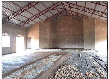
Right: Concreting a church floor - a big and costly job!
